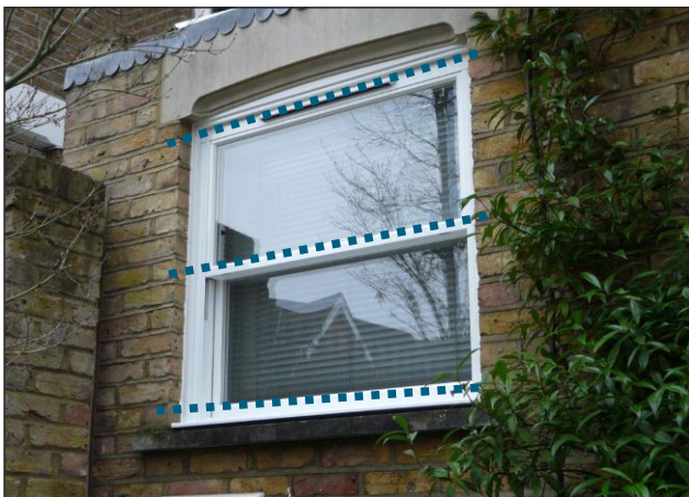
Figure 1.0: shows a traditional aluminium box sash window which has horizontal bars. Vertical Sliding secondary glazing could be made to sit behind this window discreetly.
