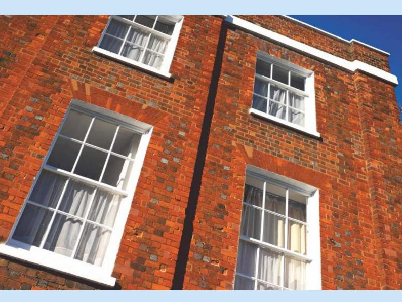
The VS Plus has a clean and simple style, that is suitable for any application, but is perfect for use in all types of modern architecture. A low maintenance alternative to wooden sash windows with the advantages of a modern thermally broken aluminium profile. The system accepts 28mm sealed units and can achieve an overall U-Value of 1.6W/m²K and a WER B rating. Ease of operation and excellent natural ventilation means that VS Plus is highly suited to high occupancy and commercial buildings.
