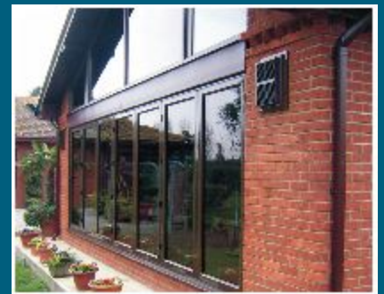
All panels closed
