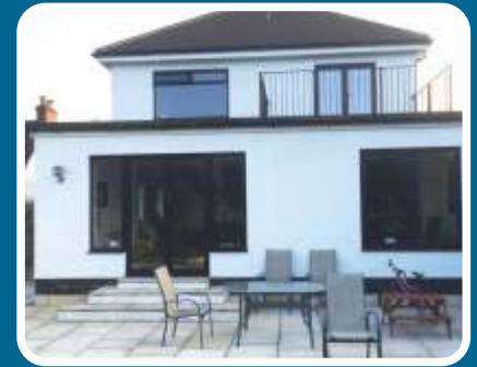
Residential Back Doors
